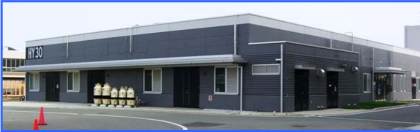
Hydrogen Technology Research Center
